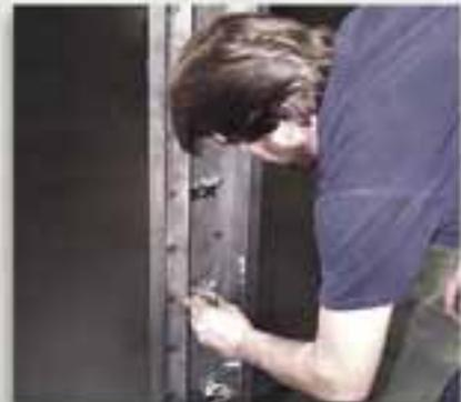
Quick release tension latches provide easy access to the finned tube core without the use of tools.
